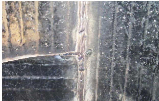
Seams between the compound steel pieces are hard welded.
